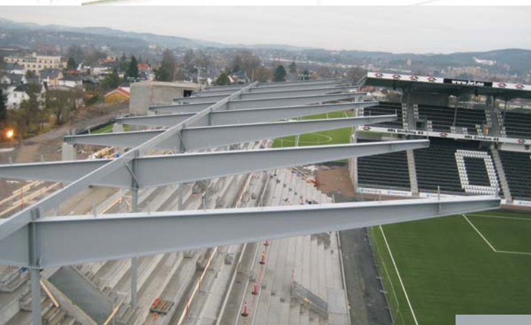
ODD stadium in Norway, 2008 – steel structures
