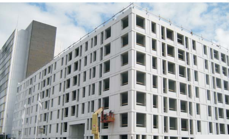
Apartment house KANALHUSENE in Copenhagen, Denmark, 2008 – prefabricated concrete constructions
