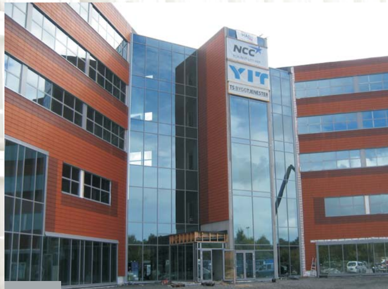
Multifunctional sports complex Trim Tower in Stavanger, Norway, 2008 - steel structures, prefabricated concrete elements
