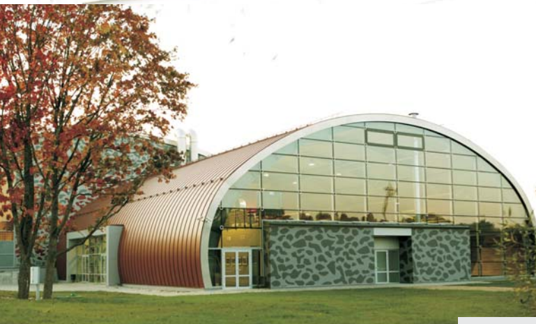
Construction of Talsu Secondary school No 2 sports hall, Talsi, Latvia, 2008
