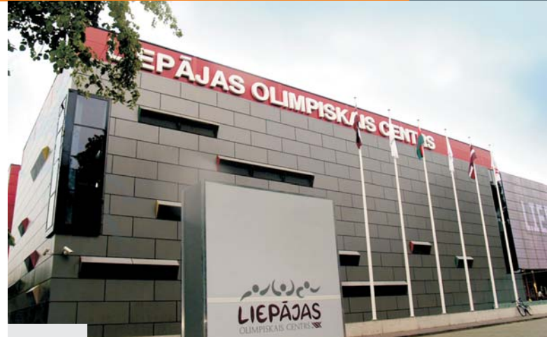
Construction of Liepāja Olympic Center 2008
