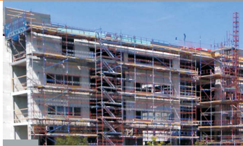
University of Uppsala Sweden, 2008 - steel structures, prefabricated concrete elements
