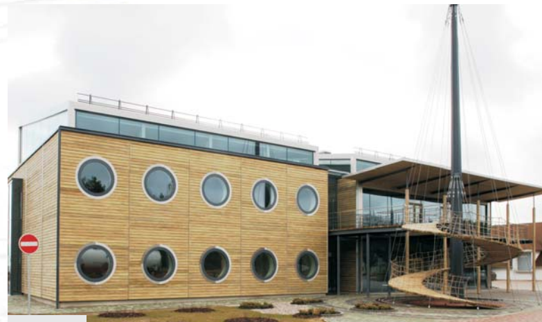
Construction of brewery Užava, Venstpils district, Latvia, 2008
